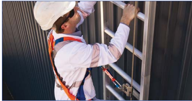
Fixed ladder with safety system, personal fall arrest system.
