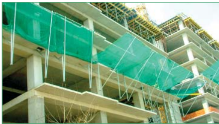
Fall arrest and safety can also be addressed with safety net systems.
