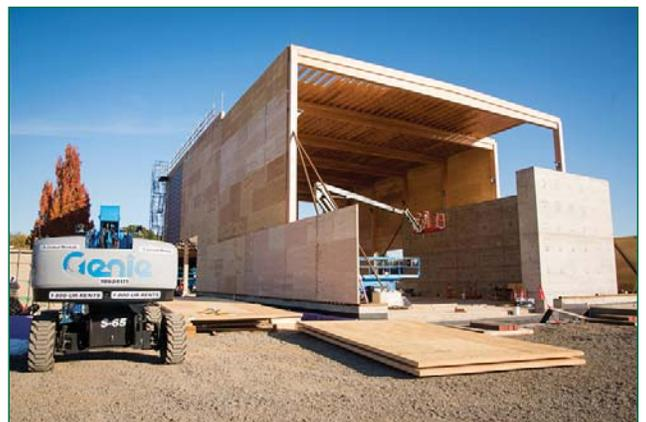
*MPP used in construction at OSU's Advanced Wood Products laboratory. Typical panel dimensions were 3" thick by 12' wide by 42' long.*
