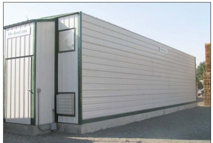
*Kiln for heat treating shipping pallets to ISPM-15 compliance.*
