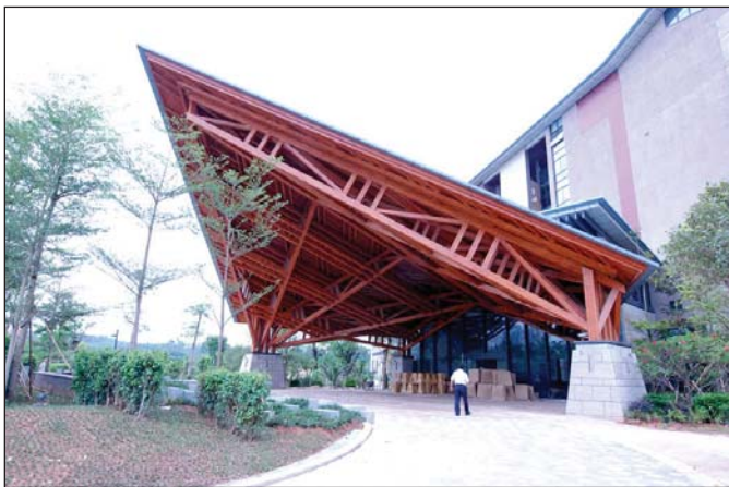
Laminated beams provide architectural flexibility as shown in the Shezhen project.
