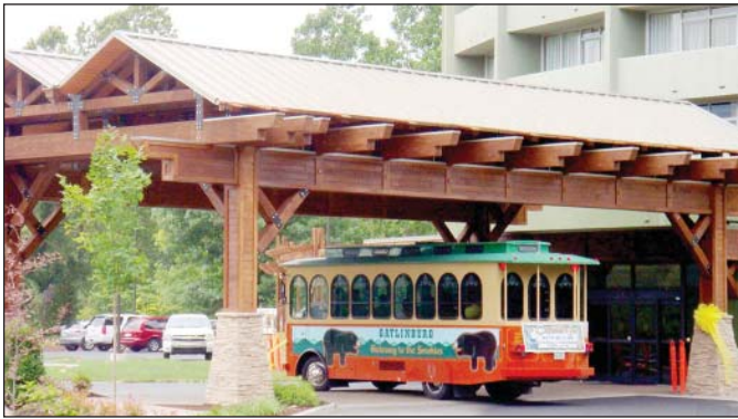
Laminated beams create an inviting entrance at the Park Vista Hotel in Gatlinburg, Tennessee.
