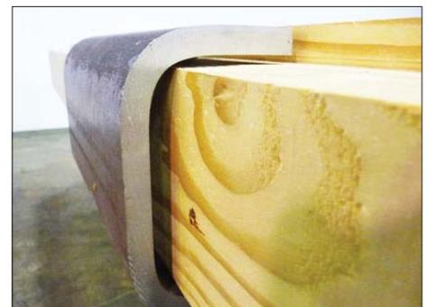
*The laminated beams are reinforced with a steel channel frame and I-beam supports longitudinally.*
