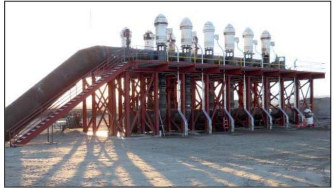
**Swaggart Brothers was the GC, using its Mechanical Division on this project. It's one of the biggest working booster stations in the Pacific NW. The project took 4 months and 14,814 man hours to complete. The booster station was built to send irrigation water to a huge number of irrigated farm circles operated by Three Mile Farms in Morrow County, Oregon.**
