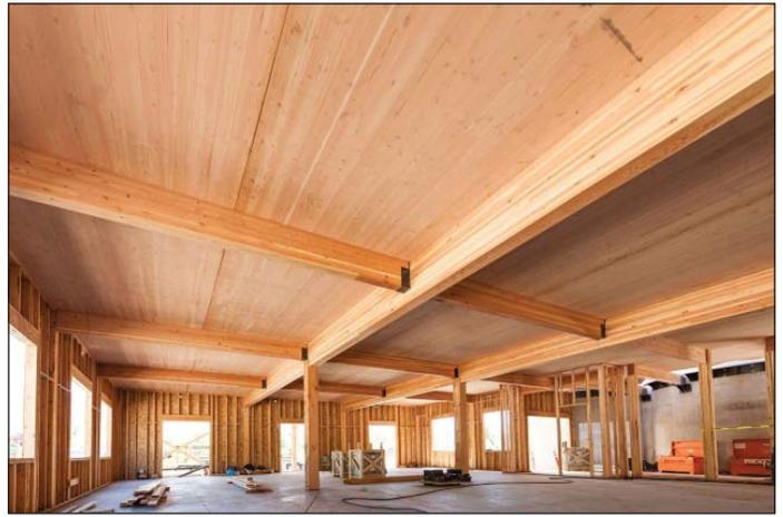
*The long wide sheet of CLT can be utilized in many building capacities, like this ceiling.*
