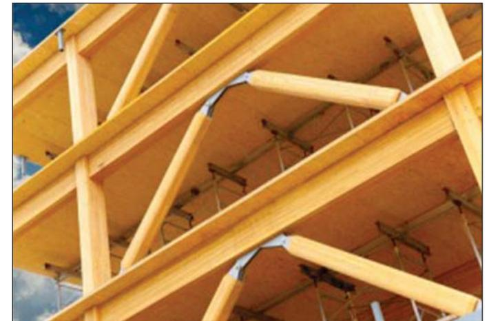
*CLT construction is five times lighter than concrete, cost competitive, fire resistant, and reduces overall construction time.*
