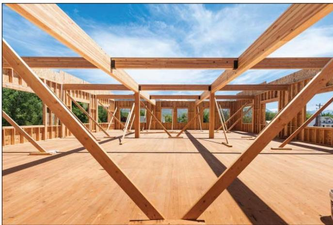
*The CLT strength makes it an ideal solution for floors over an open expanse.*
