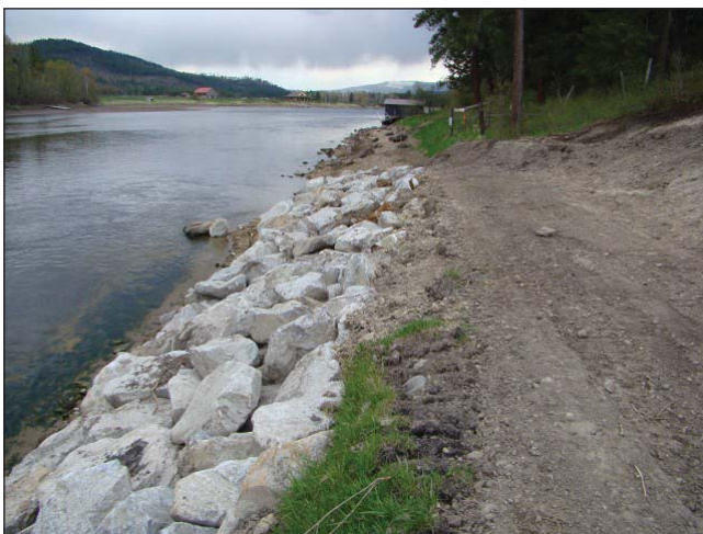
A protected shoreline is a valuable asset to water front property.
