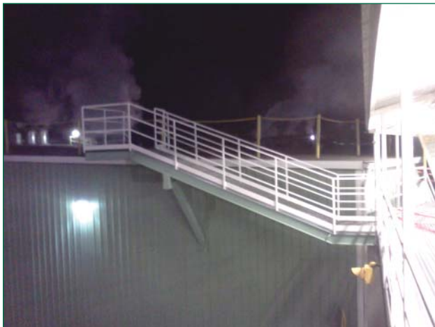
The staircase with unusual angles linking two levels at Boise Cascade in Kettle Falls, WA, was designed, manufactured and installed by Mann Industrial Contractors.
