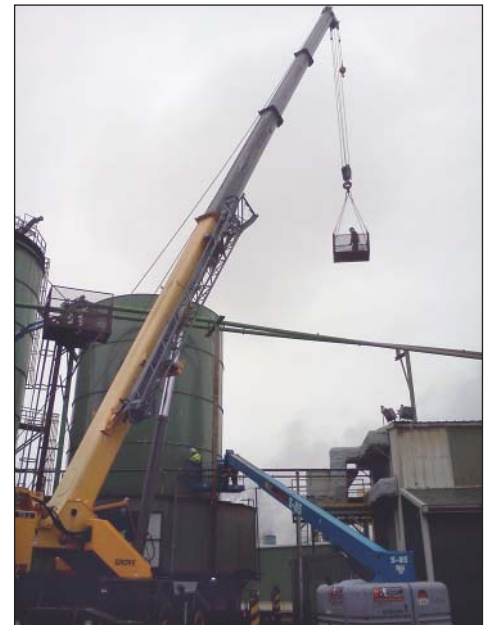
The employee in the cage is being lifted into the silo for maintenance.
