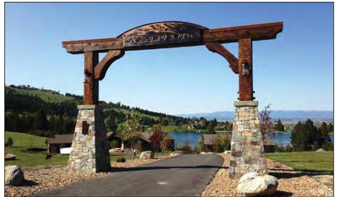
*This impressive Montana archway, built by Greg Bain and Company, features 18" X 18" Fir timbers.*
